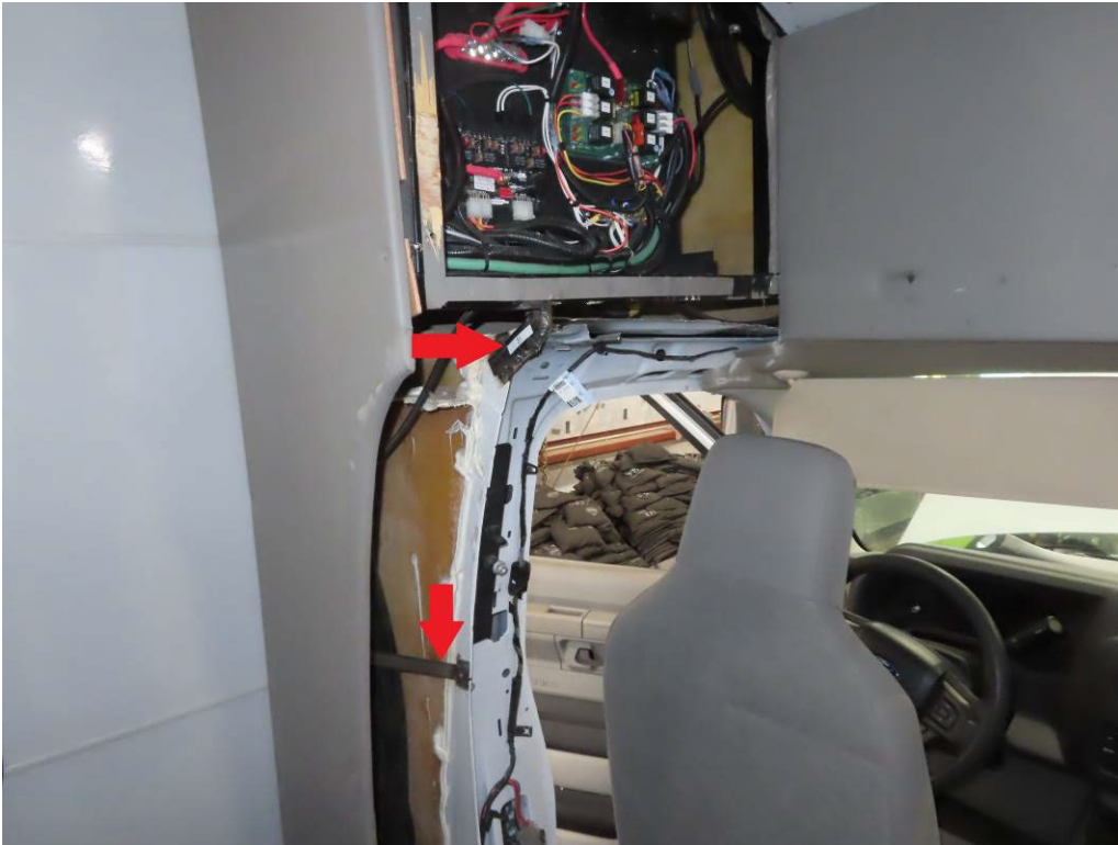
LOCATION OF CRACK #31 AND NEW SUPPORT STRAP (4,975 TEST MILES)
