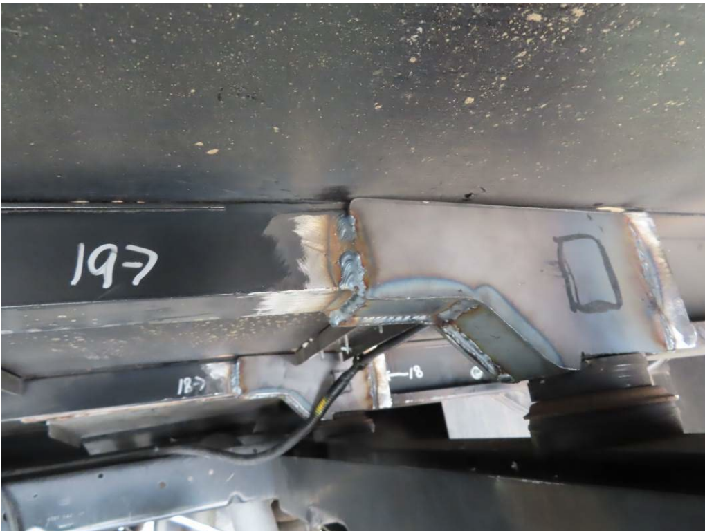
REPAIR OF CRACKS #18-2 & 19 WITH FABRICATED BRACKETS USING STEEL PLATES (2,521 TEST MILES)
