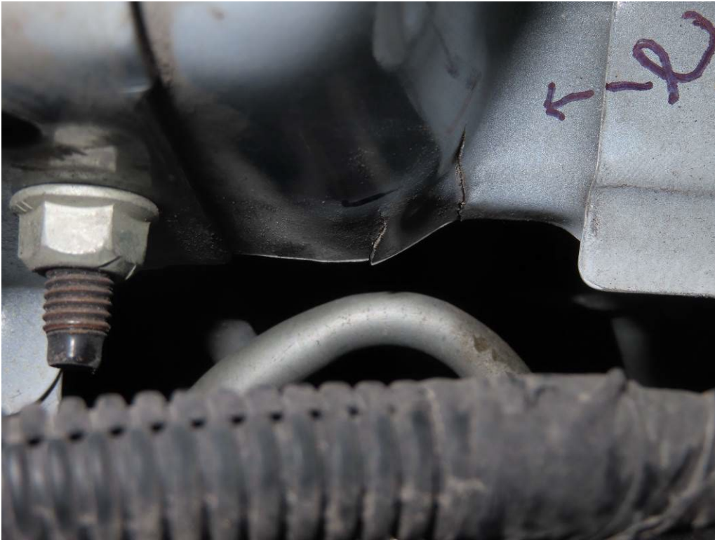
CRACK #2 – CRACKS IN BODY ABOVE THE FRAME FORWARD OF THE SUSPENSION SPRING IN THE FRONT STREETSIDE WHEEL WELL (1,123 TEST MILES)
