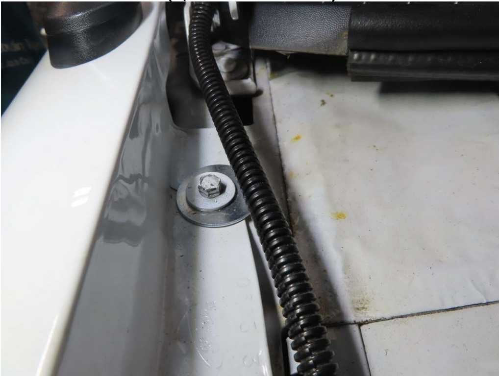
WASHER INSTALLED UNDER BOLT WHERE CRACKING ON CURBSIDE OUTER FENDER UNDER THE HOOD (4,973 TEST MILES)
