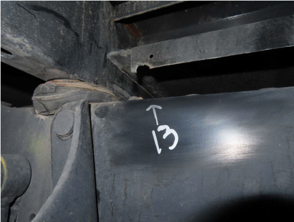
CRACK #13 – TOP OF THE CURBSIDE FRAME WHERE THE HEATSHIELD IS WELDED (1,123 TEST MILES)
