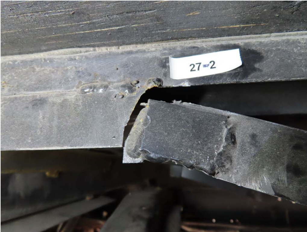
CRACK #27-2 – PREVIOUSLY REPAIRED SPLIT IN HEATSHIELD CRACKED AGAIN (7,486 TEST MILES)
