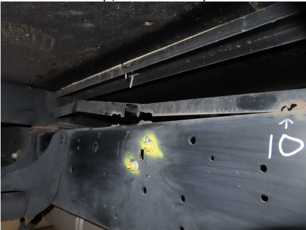
CRACKS #10, 11 & 12 – TOP OF THE CURBSIDE FRAME WHERE THE HEATSHIELD IS WELDED (1,123 TEST MILES)
