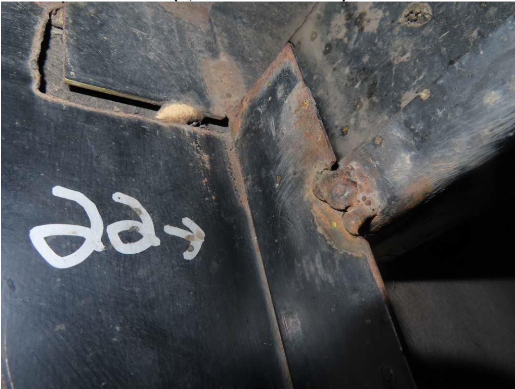
CRACK #22-2 – CROSSBEAM IN FRONT OF STREETSIDE REAR TIRES HAS A BROKEN WELD THAT WAS PREVIOUSLY REPAIRED (7,486 TEST MILES)
