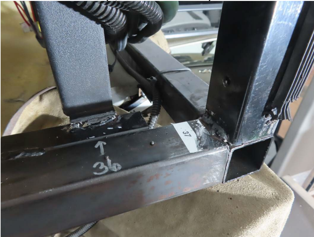
CRACK #36 & 37– VERTICAL SUPPORT AND HORIZONTAL TUBING THAT FRAMES THE FUSE PANEL (6,207 TEST MILES)
