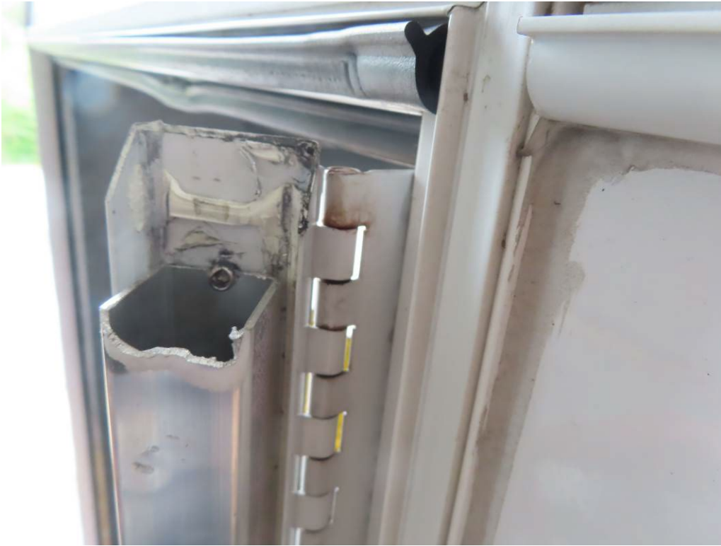
BROKEN PART OF ADA DOOR THAT FELL OFF (4,579 TEST MILES)
