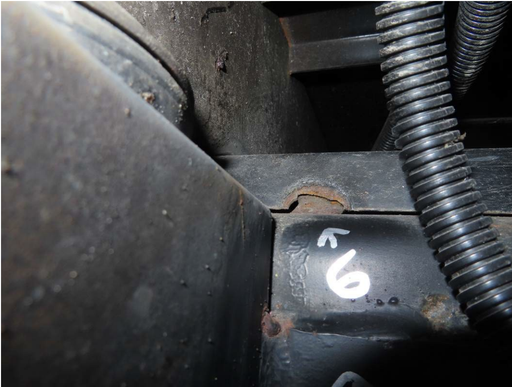
CRACK #6 – TOP OF THE CURBSIDE FRAME WHERE THE HEATSHIELD IS WELDED (1,123 TEST MILES)
